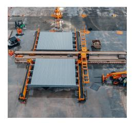
**PanelTable®** – A key to our steel erection panelization. Transforms the assembly of joist and deck for roofs and flooring.
