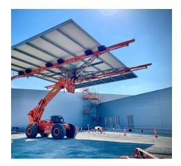
**WallMaster®** – Alows for more efficient, simpler, and safer Insulated Metal Panel (IMP) wall system installations.
