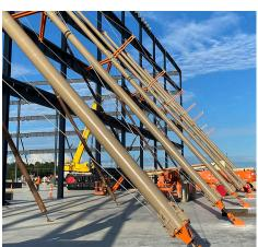
**SkyBrace®** – Provides an innovative bracing solution that ensures structural stability and improves access.
